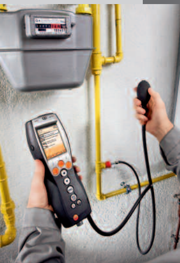
The gas pipe test
