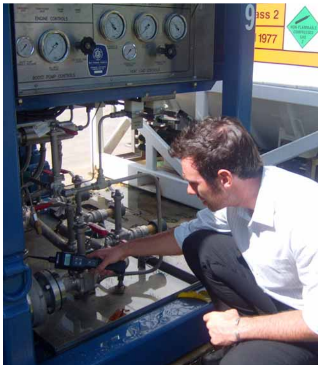
Pictured above - GasCheck 5000is being used to leak test machinery at PSL Energy Services, Singapore
