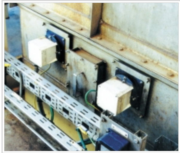
Air Duct Installation on ETAP Platform in the North Sea
